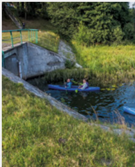
The Bytowa River Dam | Photo: AGERON Polska
