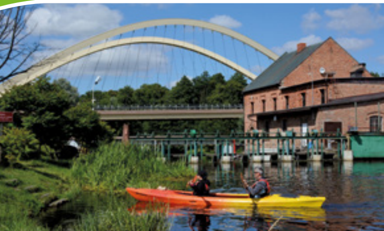
Poganice - Hydroelectric power station | Photo: L. Duchnowicz
